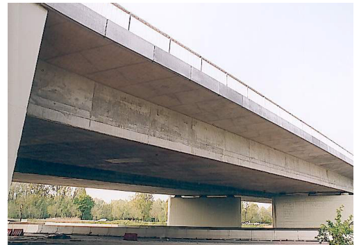
Concrete Bridge Deck
