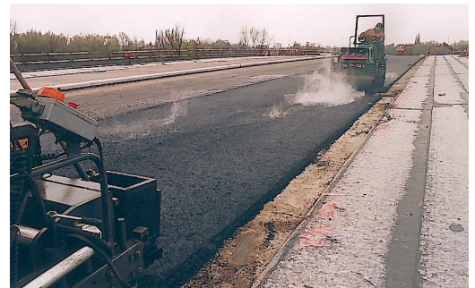
Asphalt compacting
