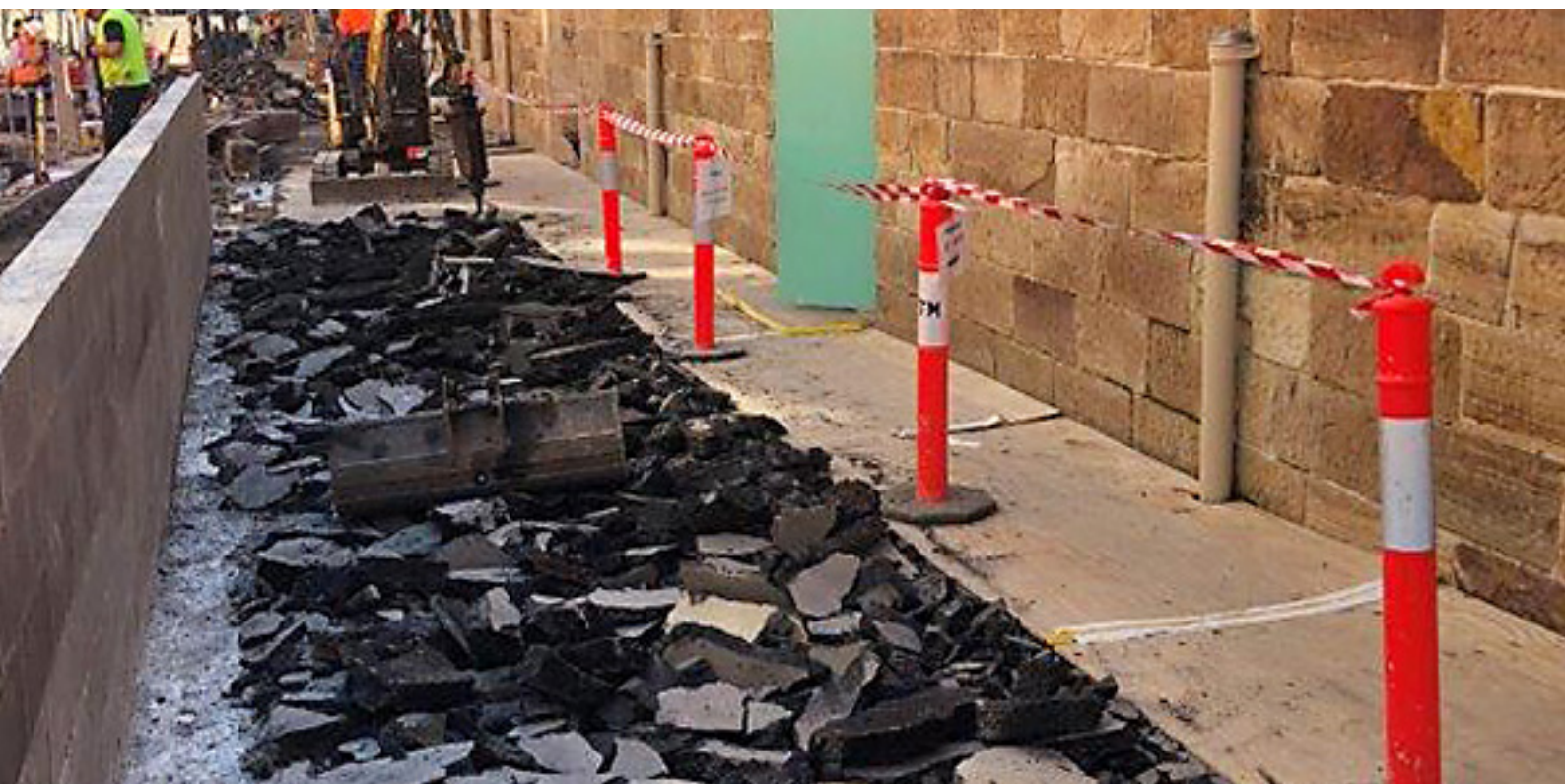
Demolishing existing asphalt
