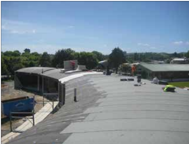
Two layer De Boer DuO membrane installation process
