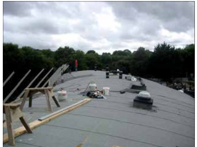
Completed DuO Landscape Capsheet, detailed around solar tubes
