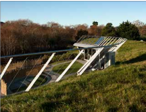
Finished gutter edge
