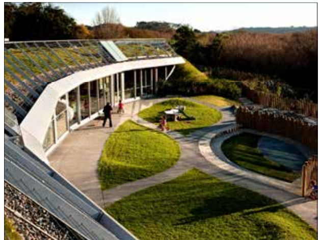
Finished gutter edge
