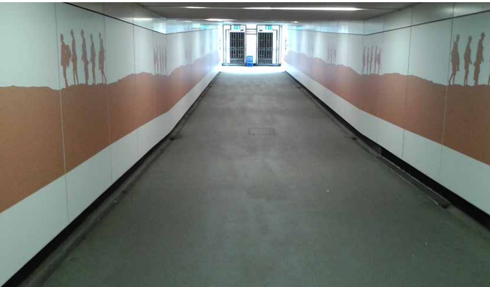
Tunnel under monument
