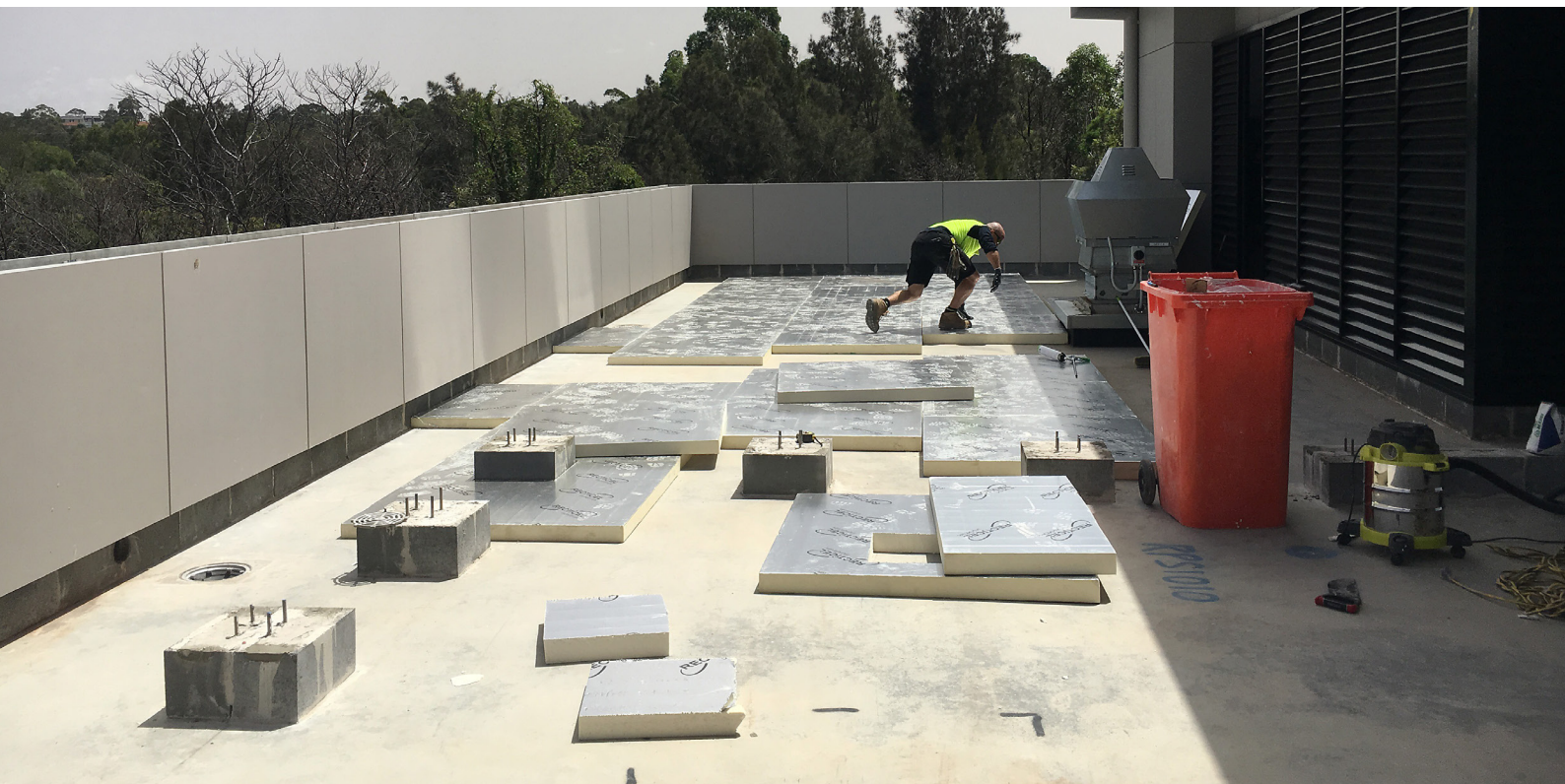
Tapered PIR Insulation installation
