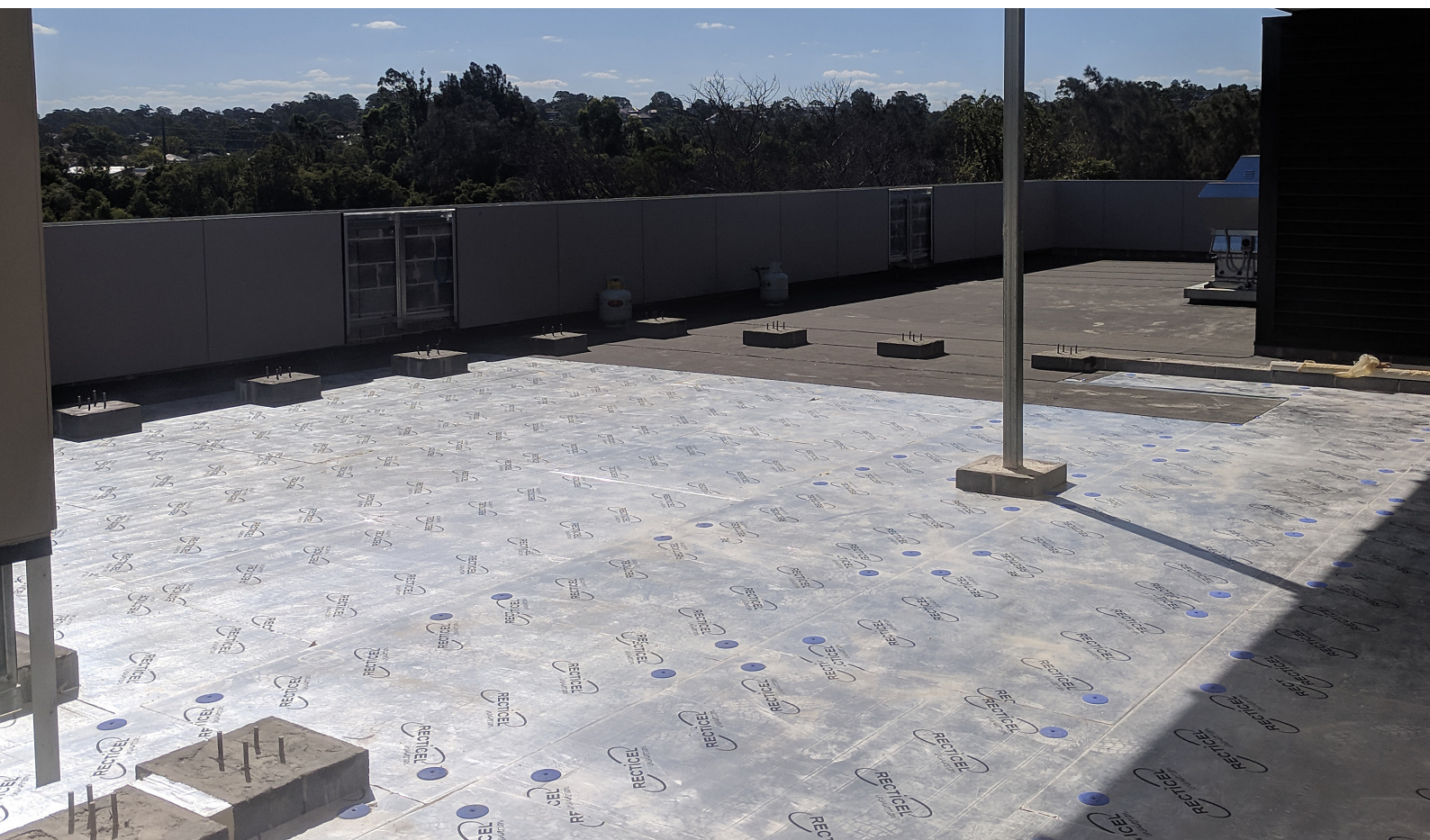
Thermal Insulation and Base Sheet
