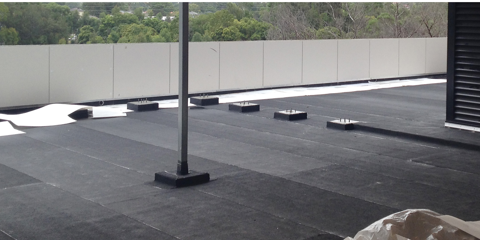
Cap Sheet installation
