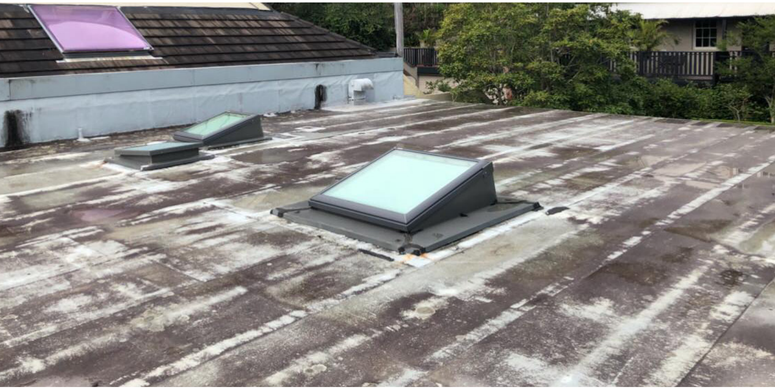
Prior to commencement
