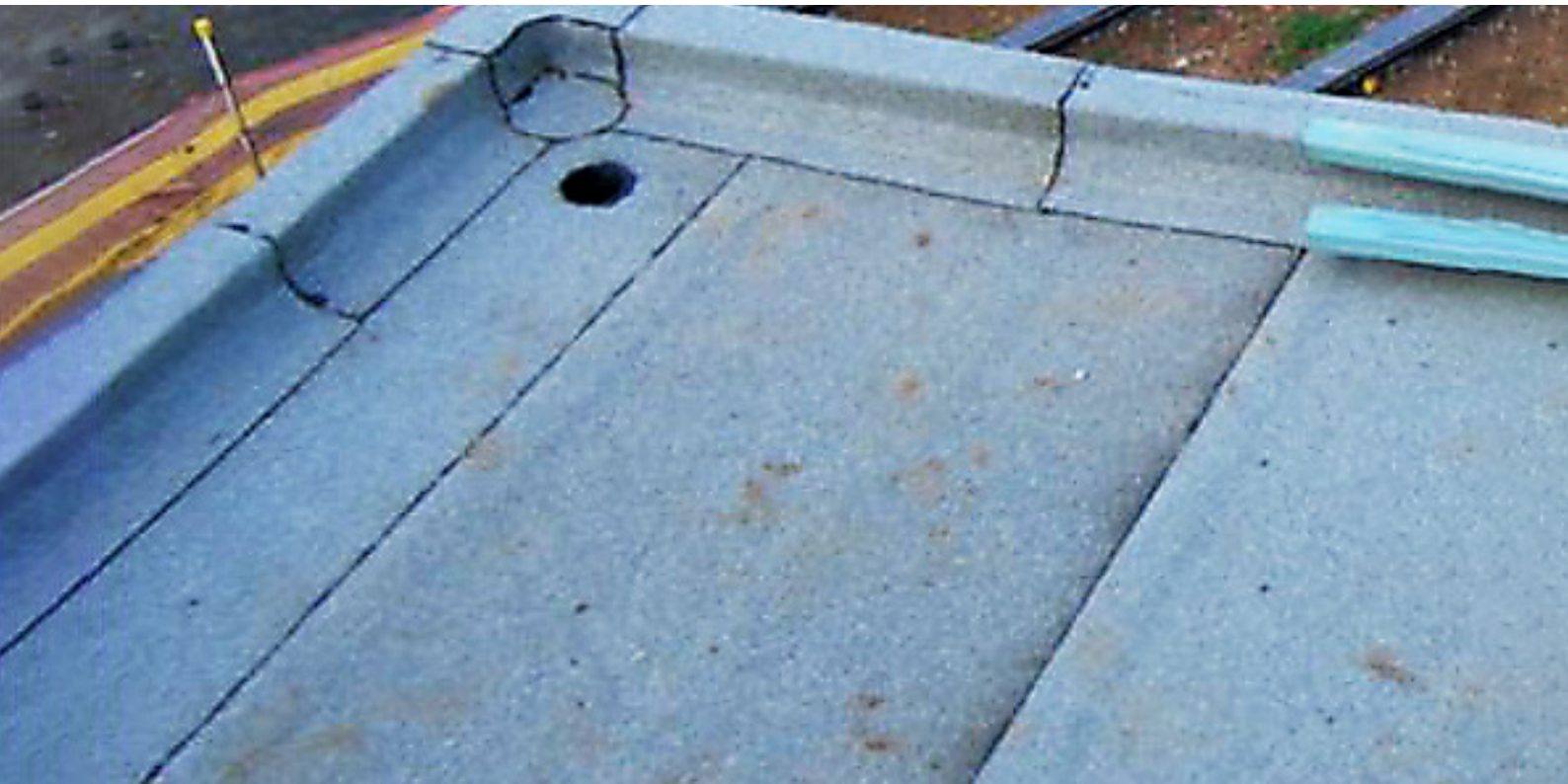
Base Sheet installation
