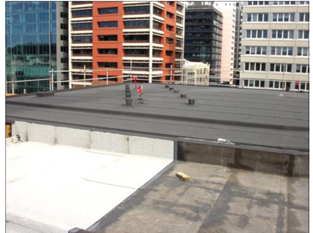
Basesheet installation
