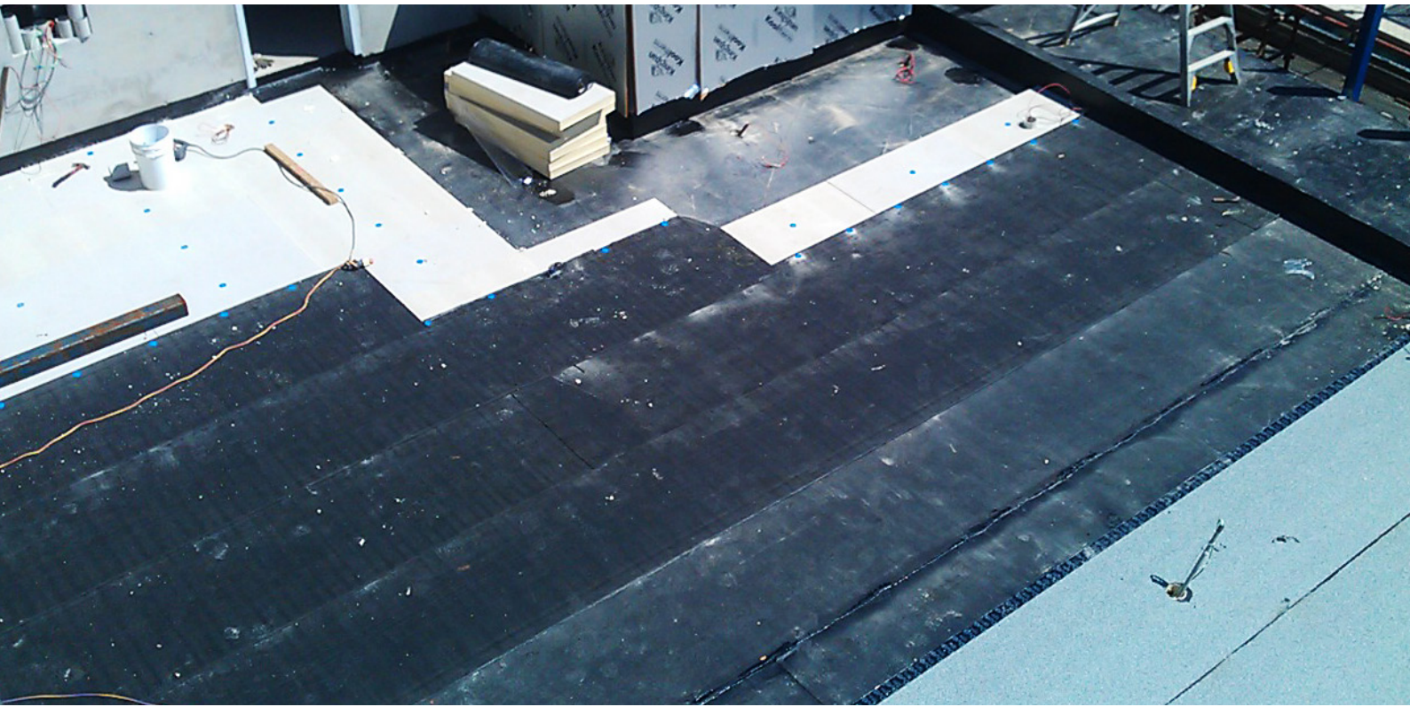
Base Sheet installation
