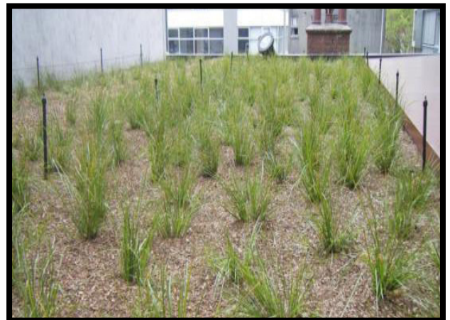
Green Roof Installation
