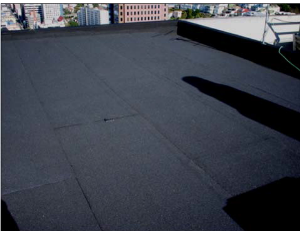
Cap sheet installation
