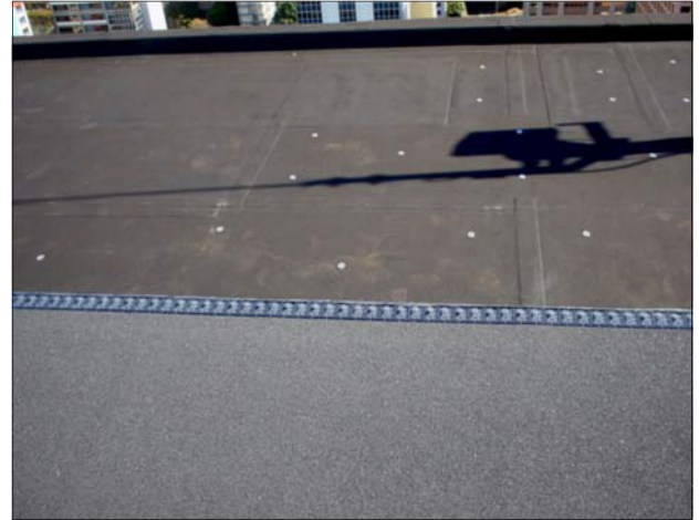
Base sheet with fasteners over Nuralite
