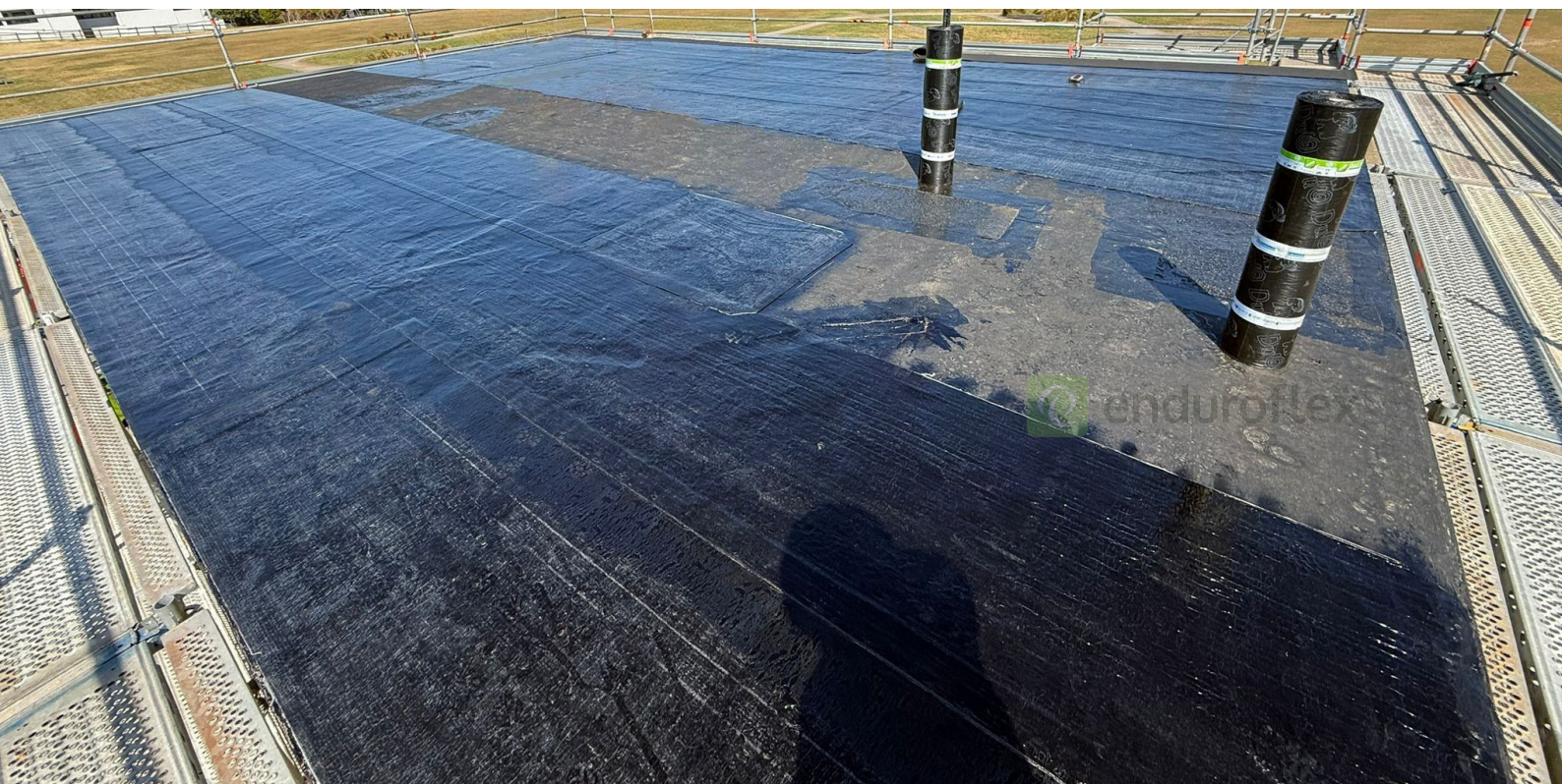
Base Sheet installation
