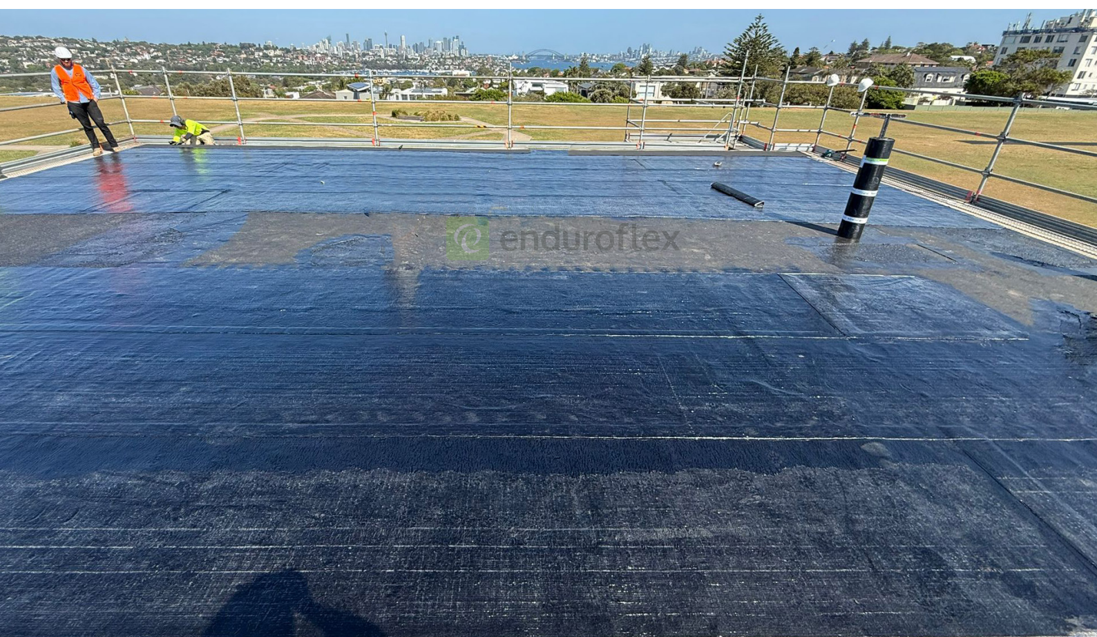
Base Sheet installation
