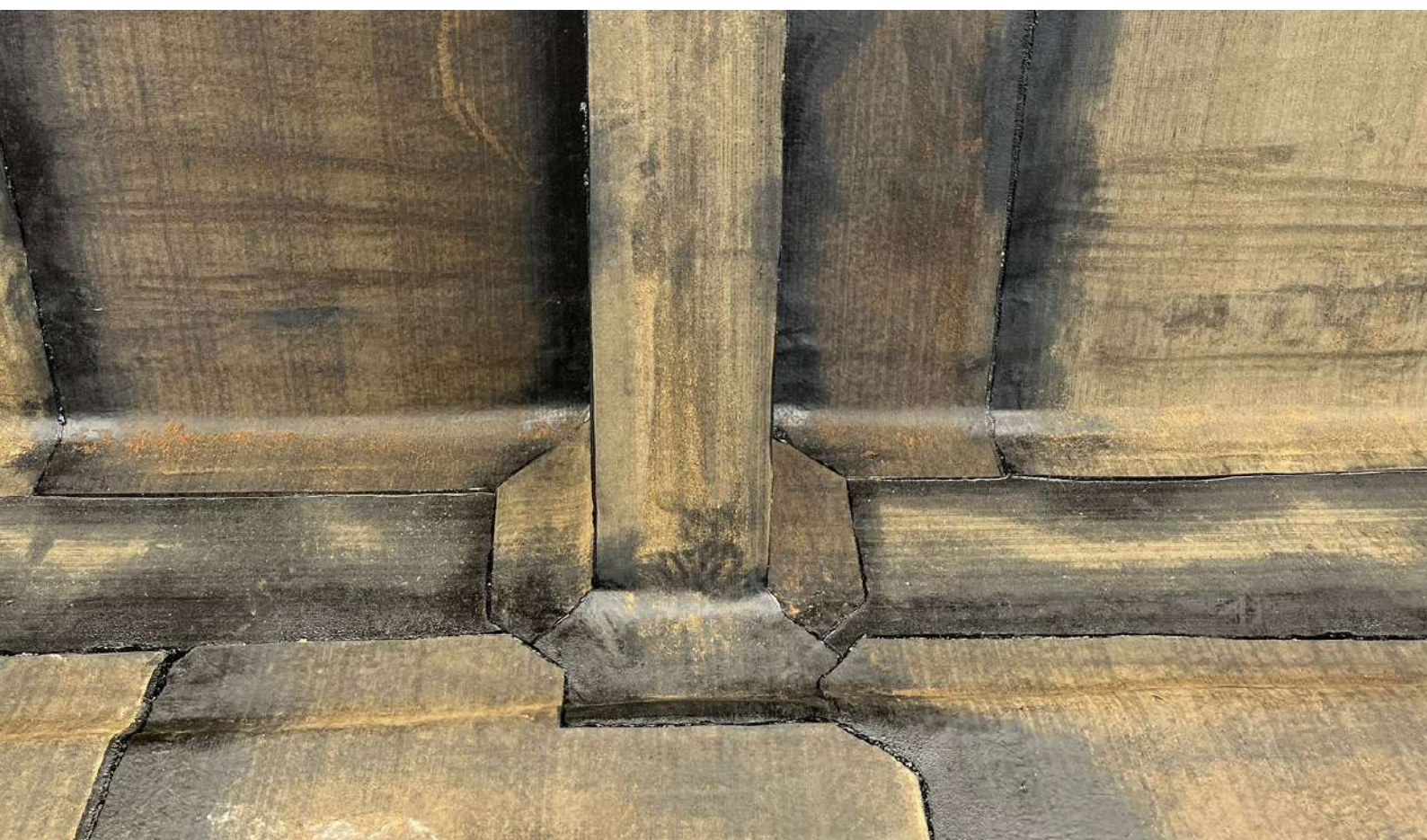
Second layer base sheet installed
