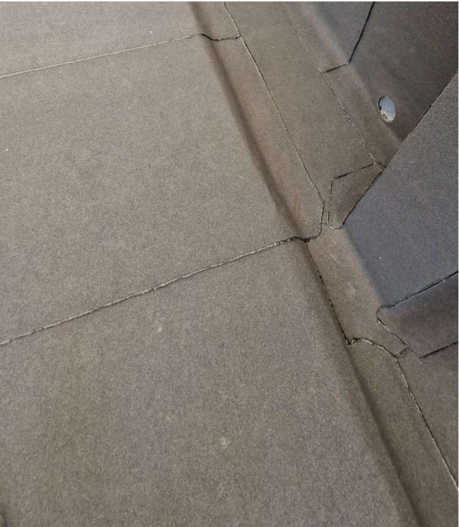
Cap Sheet installed
