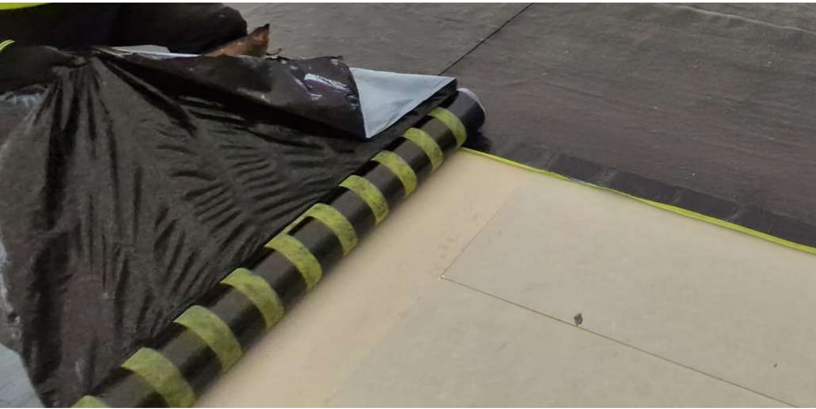
Base sheet installation on top of insulation
