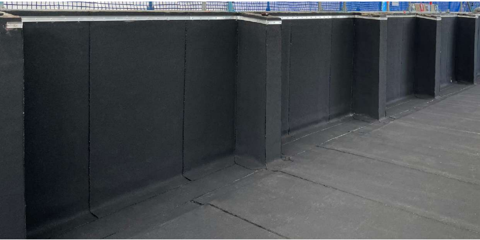
Cap Sheet installed
