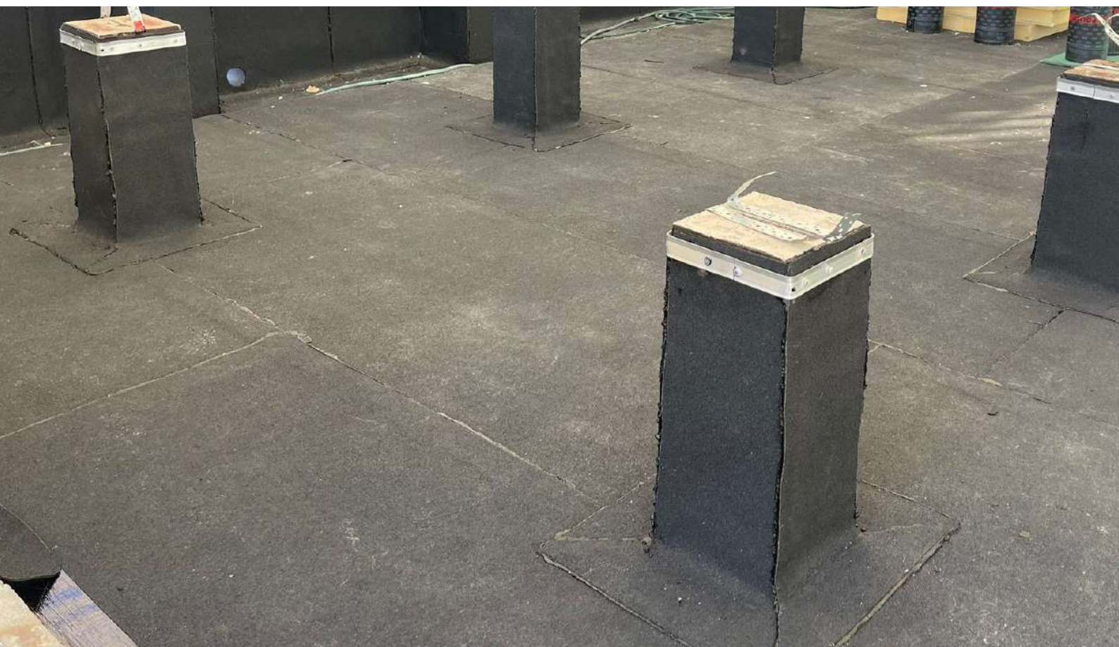
Cap Sheet installed
