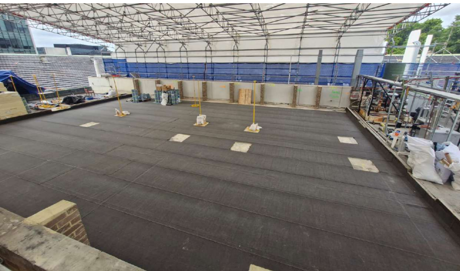
Base sheet installed
