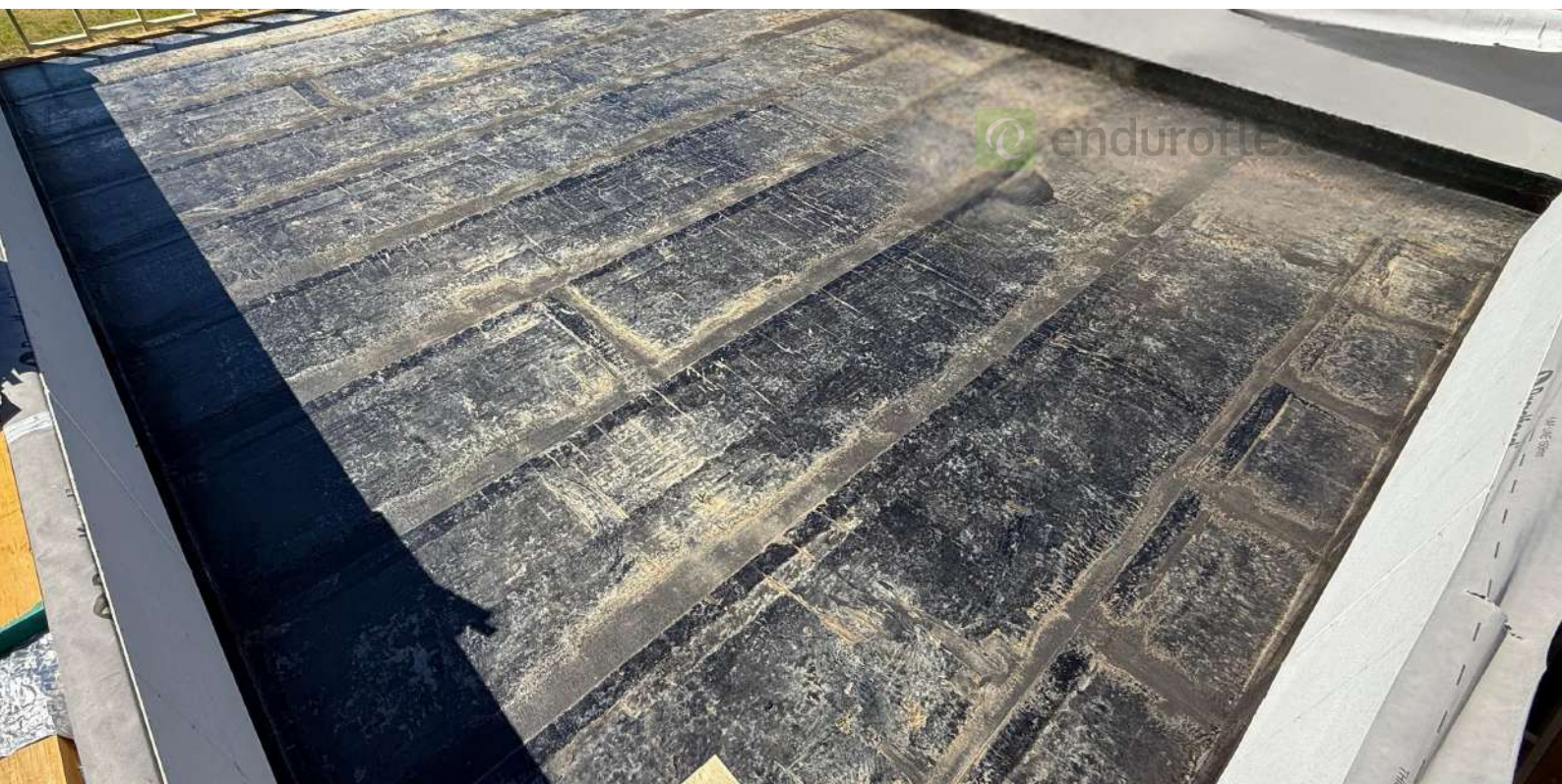
Primer and Vapour Barrier installed
