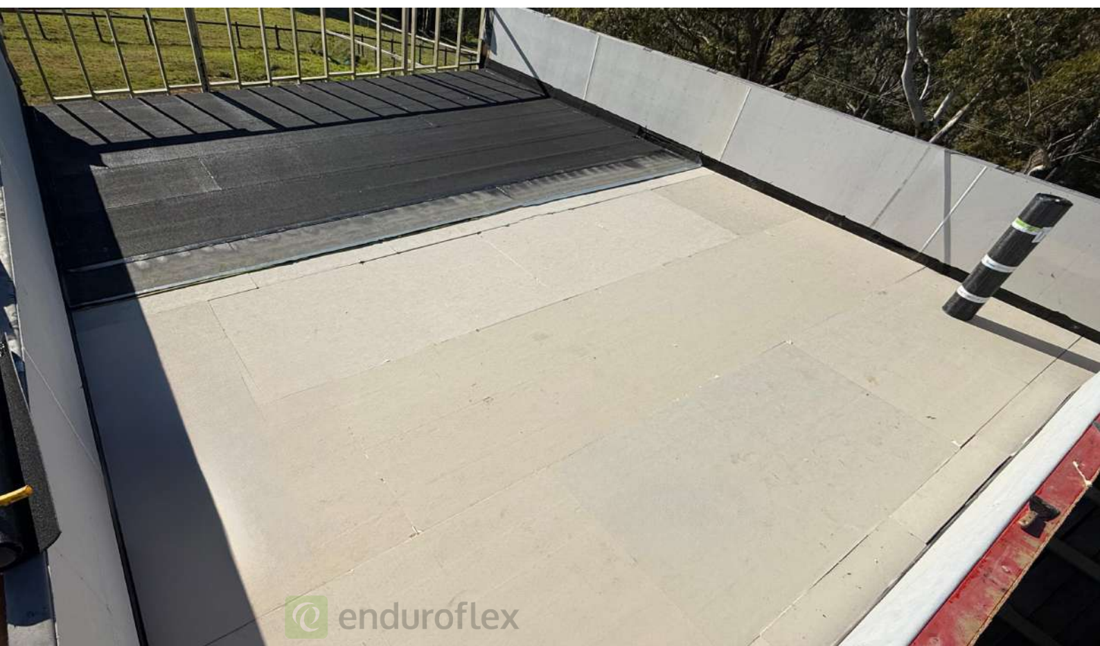
Insulation, base sheet and cap sheet
