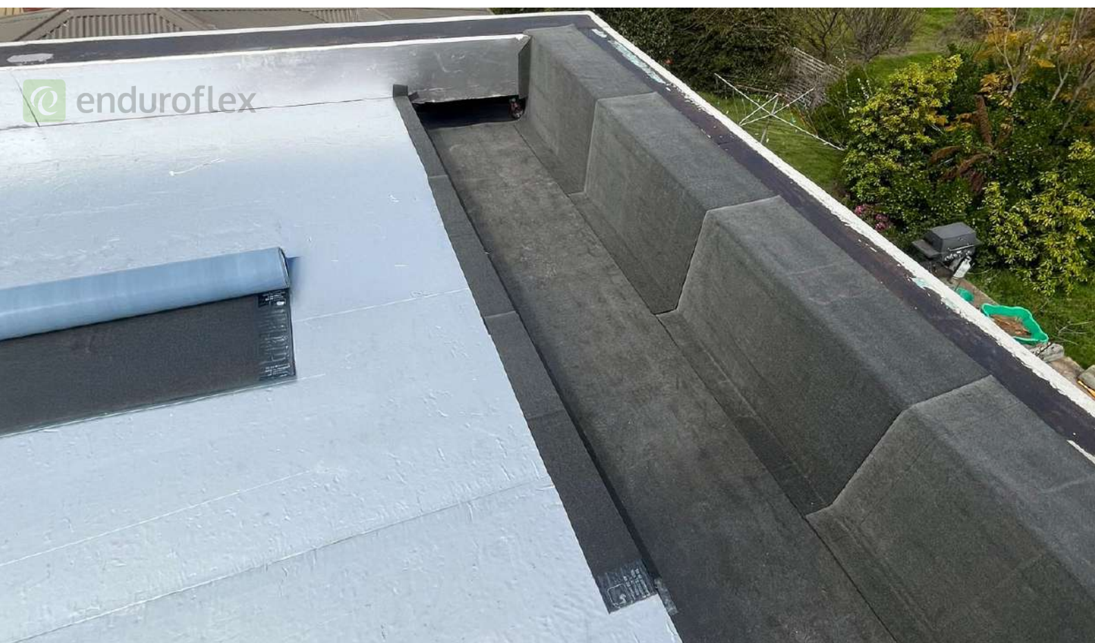
Base sheet installation
