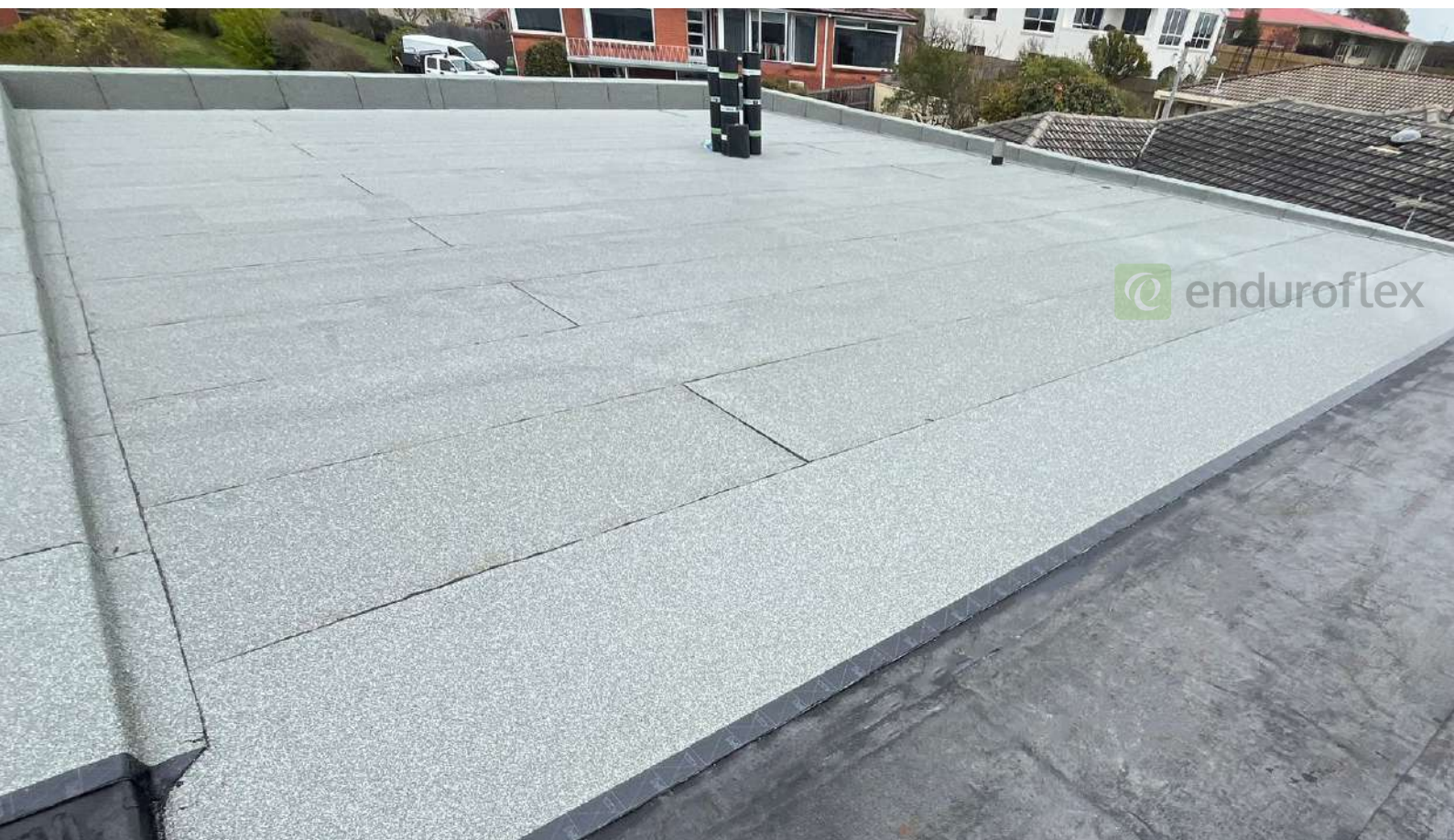
Cap sheet installation
