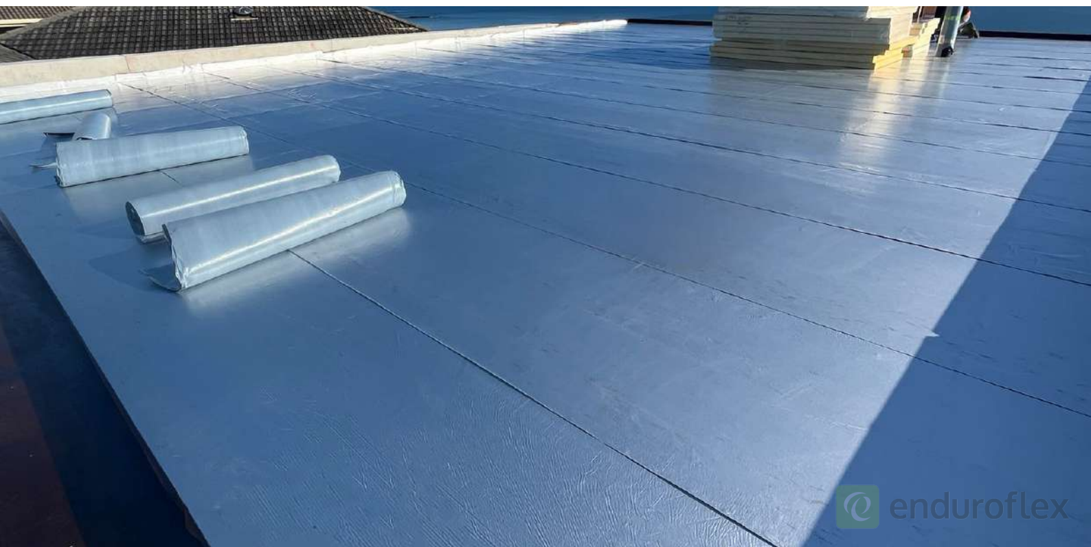
Vapour barrier installation
