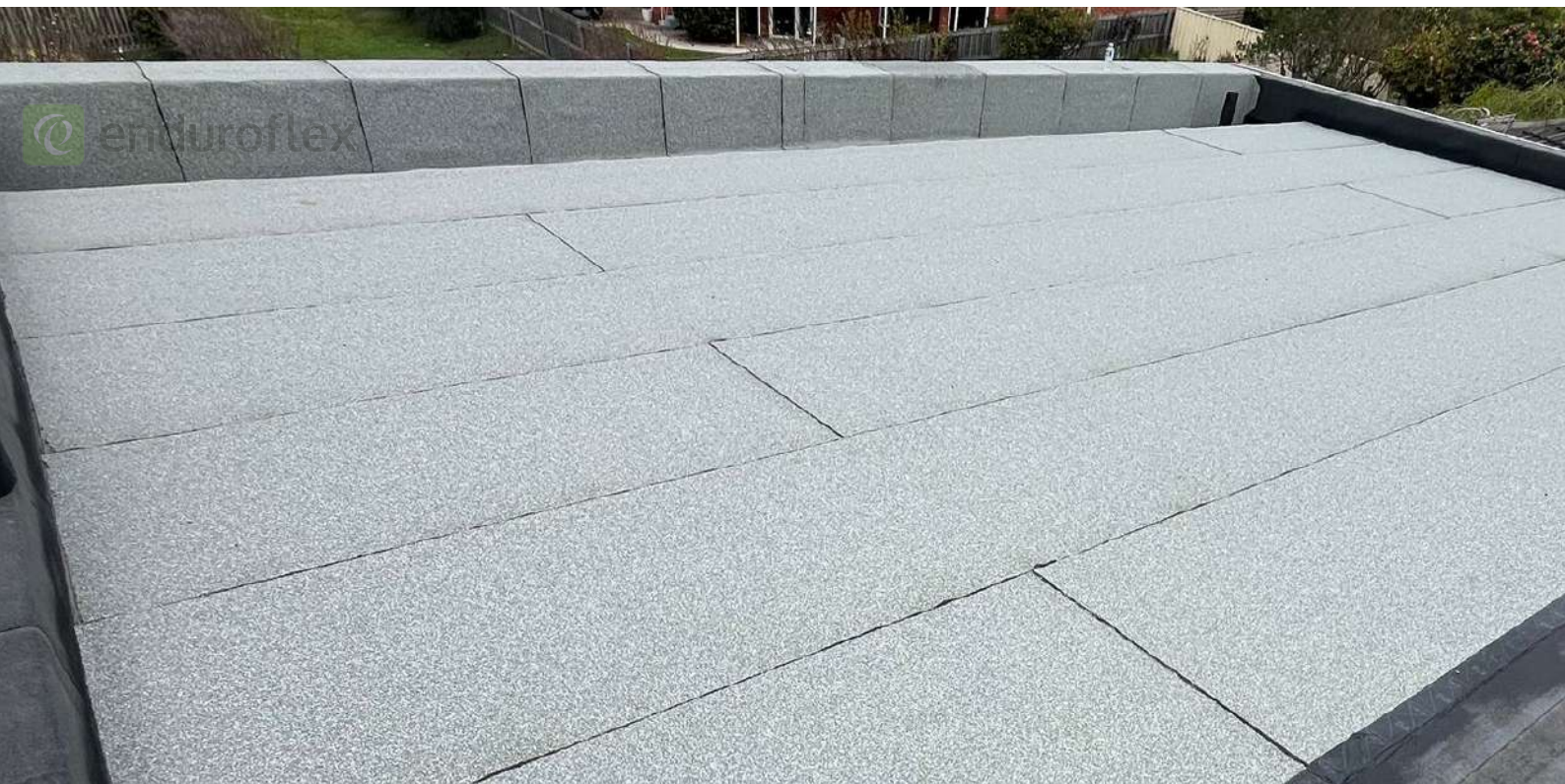
Cap sheet installation
