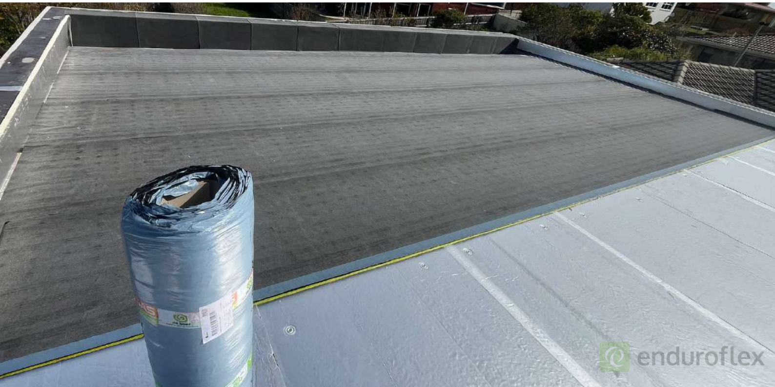
Base sheet installation
