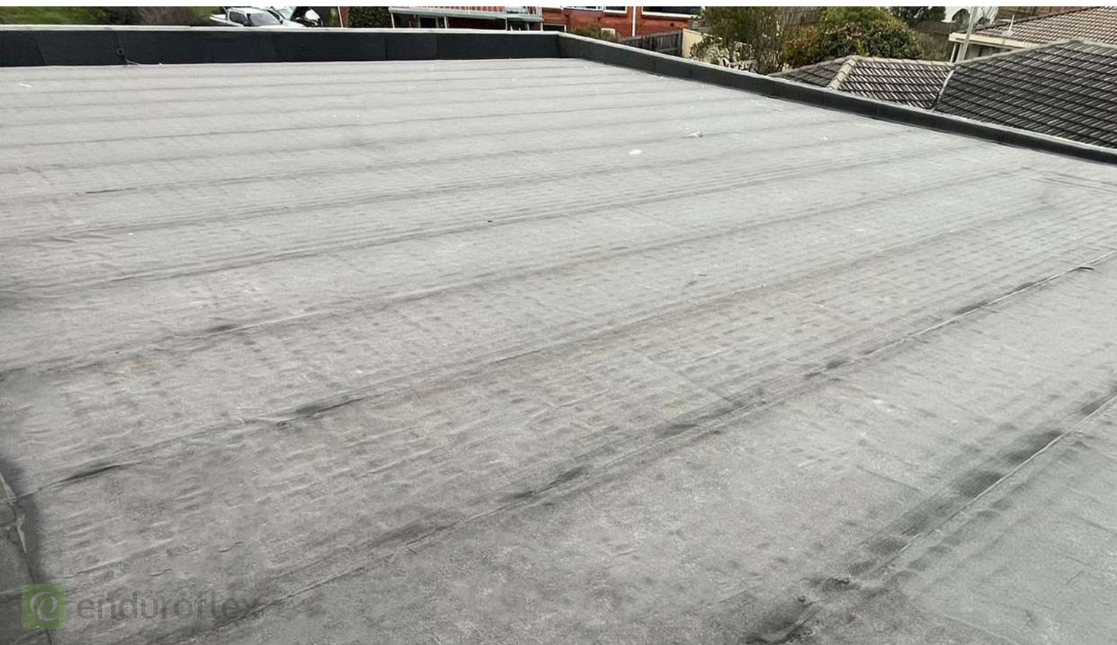
Base sheet installed
