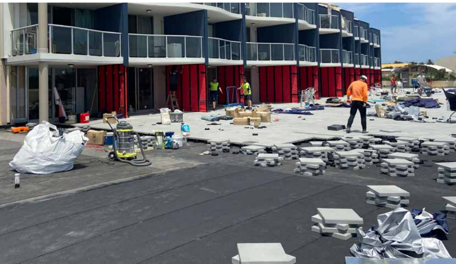
Pavers and support pads
