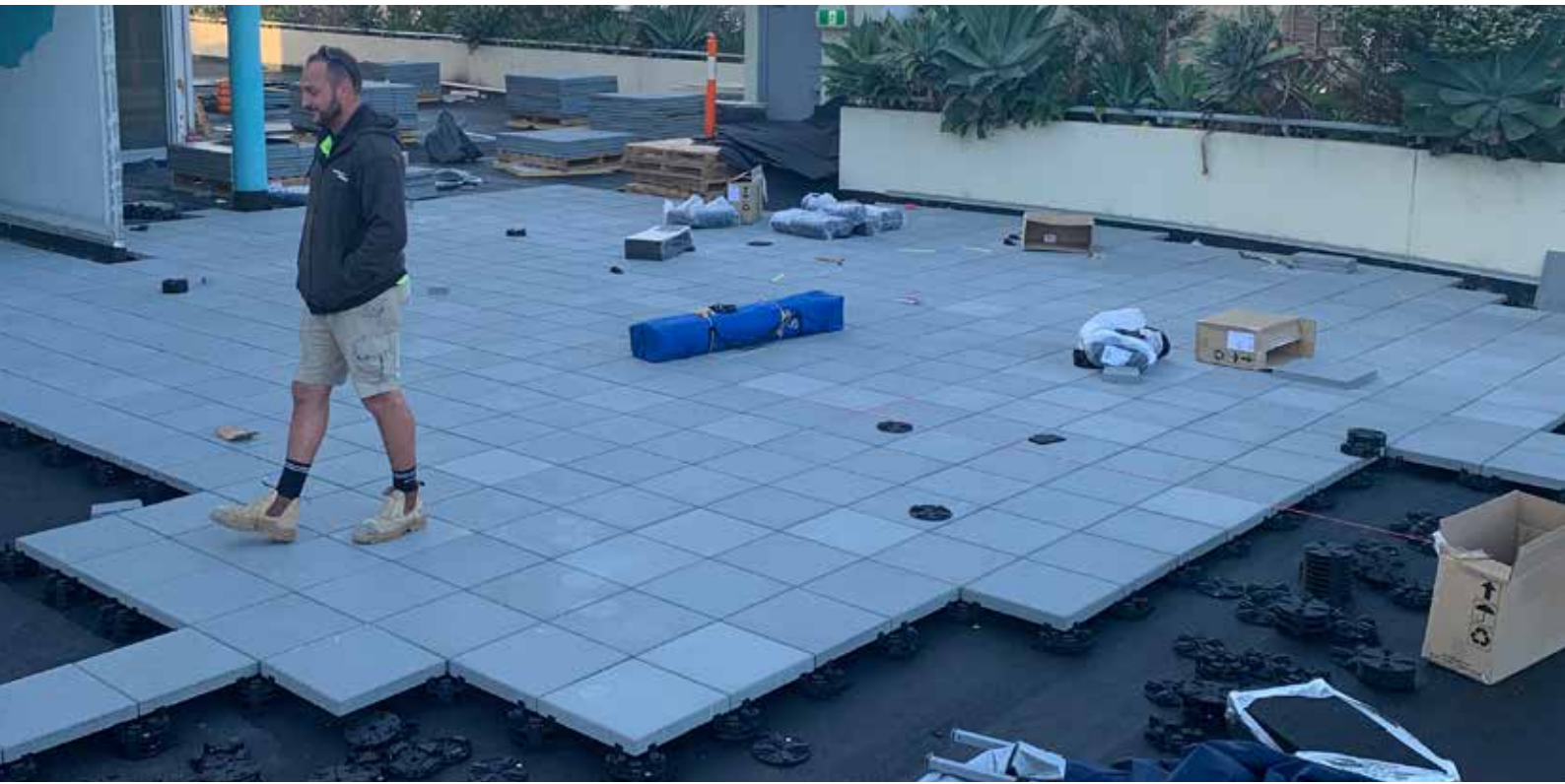
Pavers and support pads
