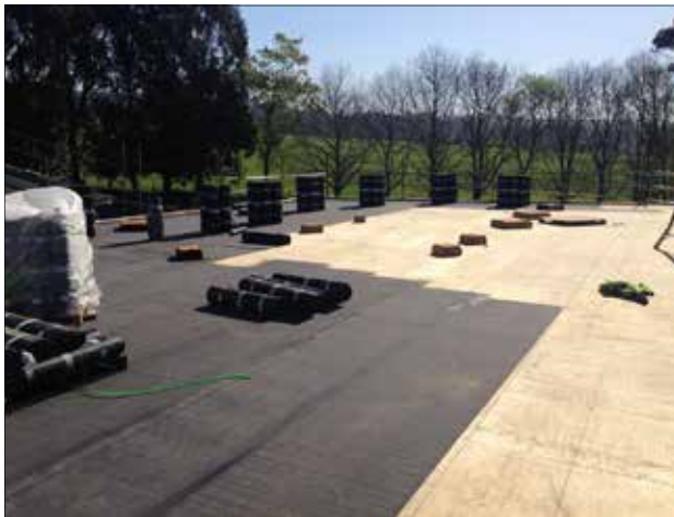
Vapour barrier and plywood substrate
