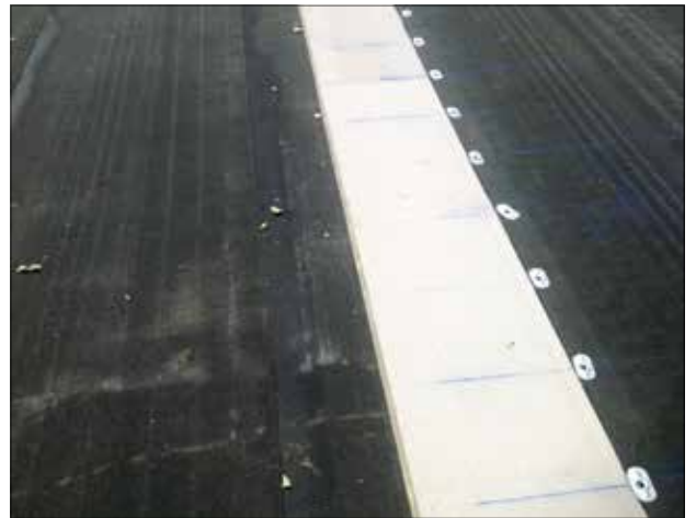
Vapour barrier, PIR board, mechanically fastened basesheet
