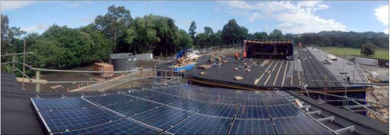
View showing several different stages of construction
