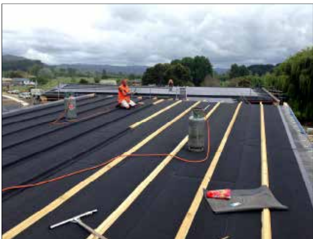
Capsheet and batten installation
