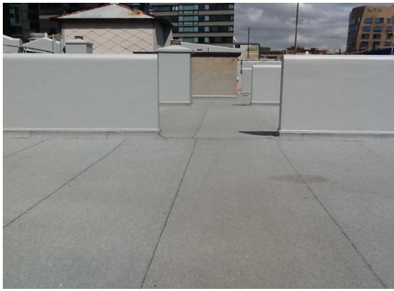
Capsheet Installation finished
