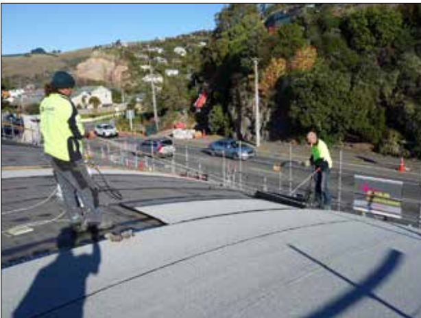
Installation of Duo cap sheet
