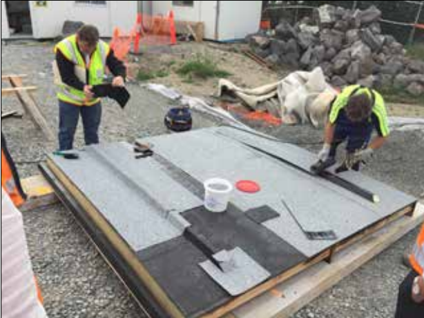
Preparation of the Duo mock roof
