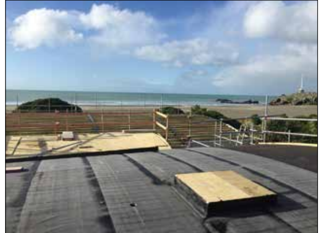
Installation of the Duo basesheet over plywood
