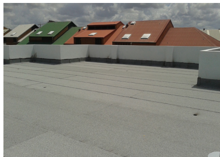
Henderson Road - Alexandria NSW
